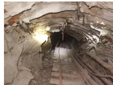
Fig.1 Large deformation of surrounding rock
