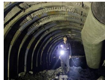
Fig.2 Field application of confined concrete support
